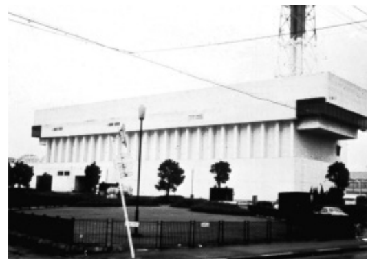
Garbage Incinerator Facility
