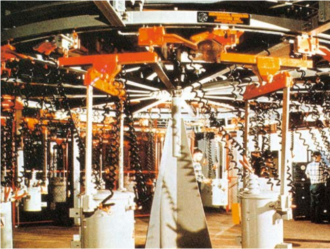
Power-and-free conveyor system
