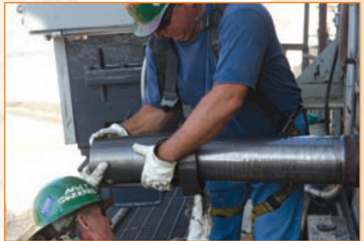
Tapered bushing with the Falk V-Class drive will make it easier to remove and eliminate the need to destroy components, as with the previous drives.
