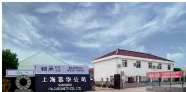
Esterno laboratorio External view of laboratory
